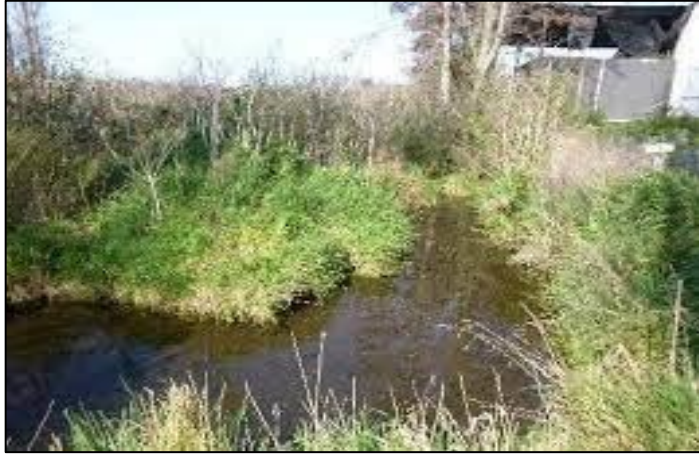
Water logging due to seepage
