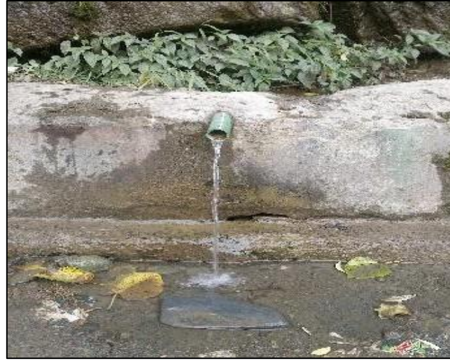
Springs with piped outlet
